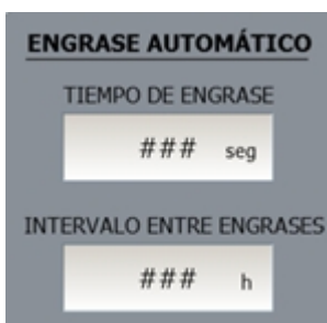
CONTROL WINDOW OF AUTOLUBRICATION SYSTEM
